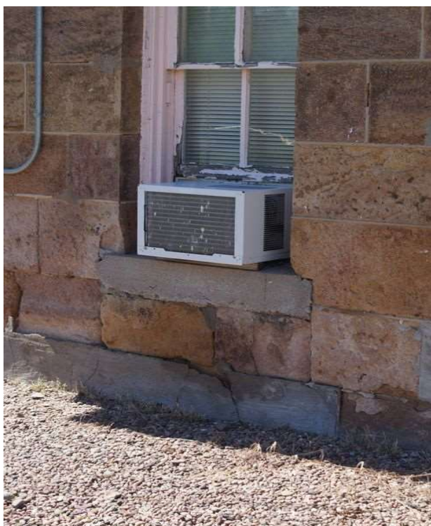
003: Fort Dodge Officers House ca. 1867 (KHRI: 057-1821-00005). North elevation window and a replaced, concrete window sill; looking southeast.
