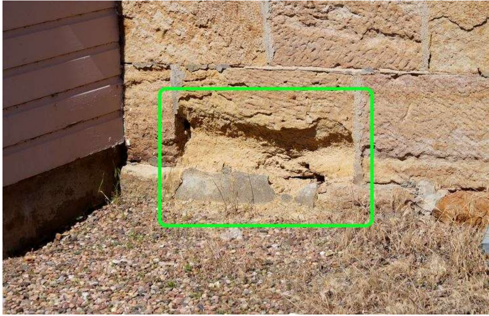
004: Fort Dodge Officers House ca. 1867 (KHRI: 057-1821-00005). East elevation at ground level; looking west. Approximately one-half of the stone's face has spalled away. Note concrete in area.
