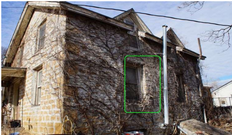
002: Mitchell, Thomas W., House (KHRI: 139-365) East elevation; looking northwest. Wall is bowing outward just right of the left window. Here the sun is shining on the protruding portion [circled in green] of the wall and to the left of the vent pipe. Note also the amount and size of the vines growing on the house in this area.
