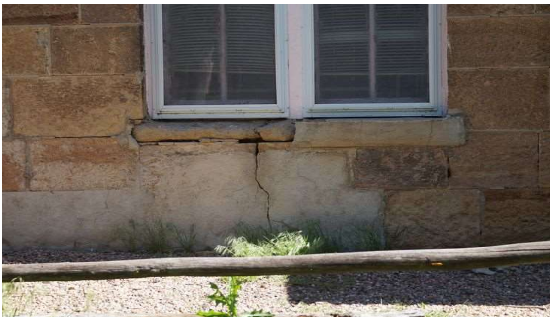
002: Fort Dodge Officers House ca. 1867 (KHRI: 057-1821-00005). South elevation windows; looking north. Concrete filled under window with damaged sill.
