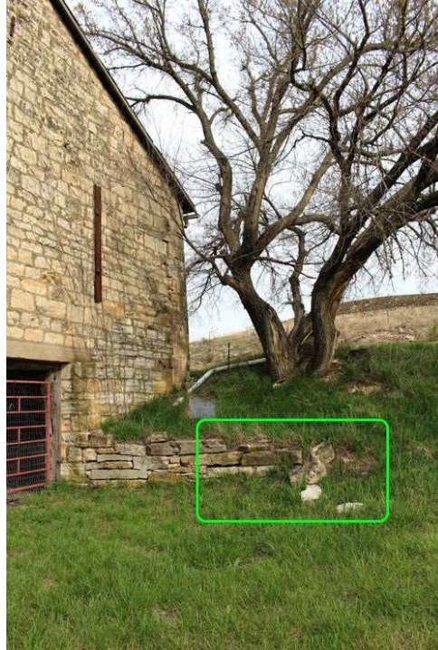
005: Morris: Big John Farm Limestone Bank Barn (KHRI: 127-0000-00040) Looking north at the east elevation's north wing-wall. Area of green box indicates the wall being overtaken by dirt and hydrostatic pressure moving the stones. Note large tree growing too close to the barn and wing-wall.
