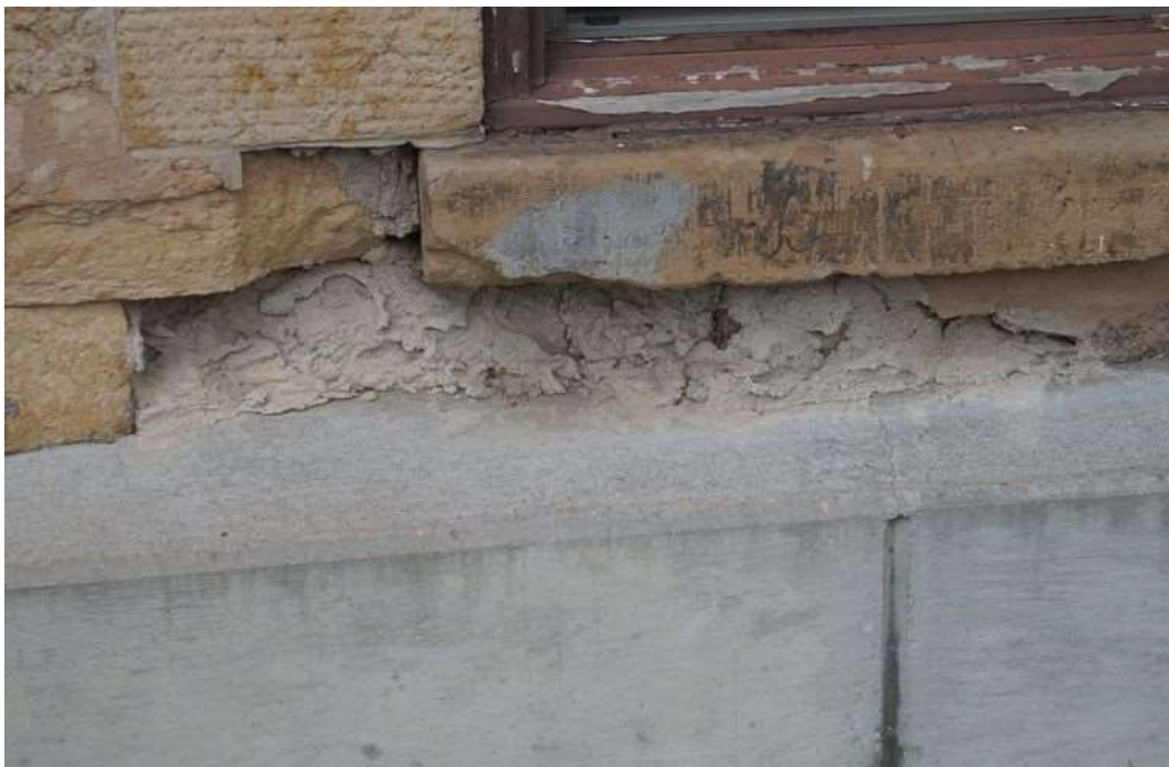
005: Fort Dodge Enlisted Men's Barracks ca. 1867 (KHRI: 057-1821-00003). South barracks east elevation, typical window sill and spalled sandstone just above the concrete/gunite; looking west.
