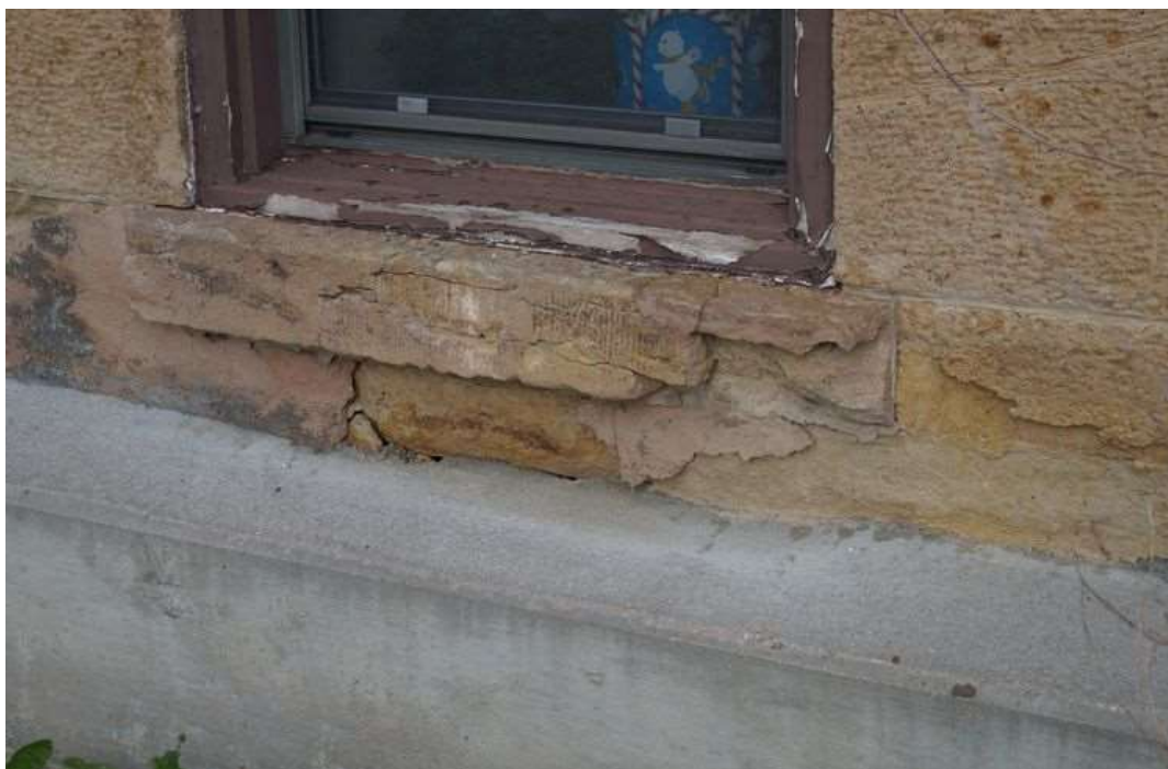
006: Fort Dodge Enlisted Men's Barracks ca. 1867 (KHRI: 057-1821-00003). Sandstone window sill and concrete/gunite application on east elevation of south barracks; looking west.
