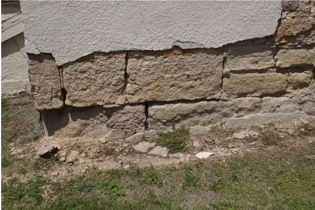
004: Fort Dodge Army Quartermaster Building ca. 1867 (KHRI: 057-1399). East elevation at southeast corner of building; looking west. Note bottom corner stone has totally spalled.
