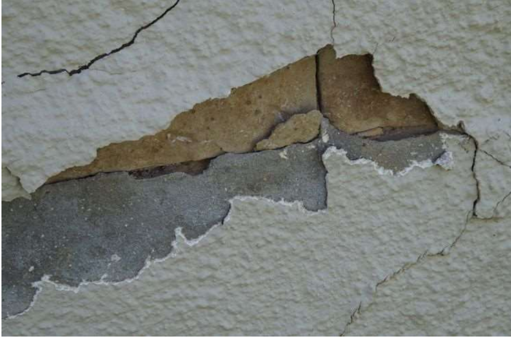
002: Fort Dodge Army Quartermaster Building ca. 1867 (KHRI: 057-1399). West elevation; looking east. Note the application of concrete first under the second attempt with stucco.
