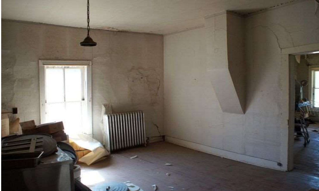
007: Fort Dodge Junior Officers' Quarters ca. 1870 (KHRI: 057-1426). Interior, first-floor east half of Junior Officers Quarters; looking southeast in the northeast room. The wall with the window is the area of water intrusion. Note plaster above register and to the right of the window.
