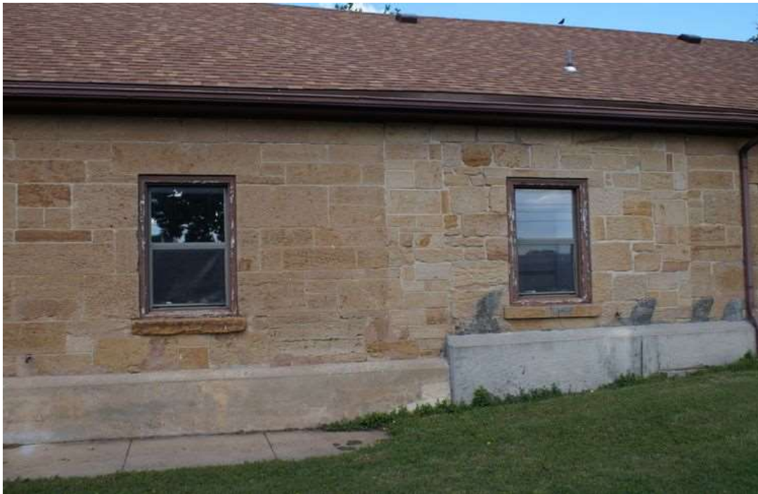
004: Fort Dodge Enlisted Men's Barracks ca. 1867 (KHRI: 057-1821-00003). East elevation of south barracks; looking west. Note two different applications of concrete/gunite to lower areas of the walls.
