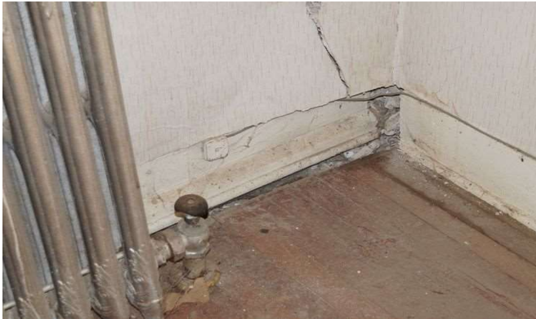
008: Fort Dodge Junior Officers' Quarters ca. 1870 (KHRI: 057-1426). First-floor, east side of Junior Officers Quarters; water damage and settling of the floor from the wall in the northeast corner of the northeast room.
