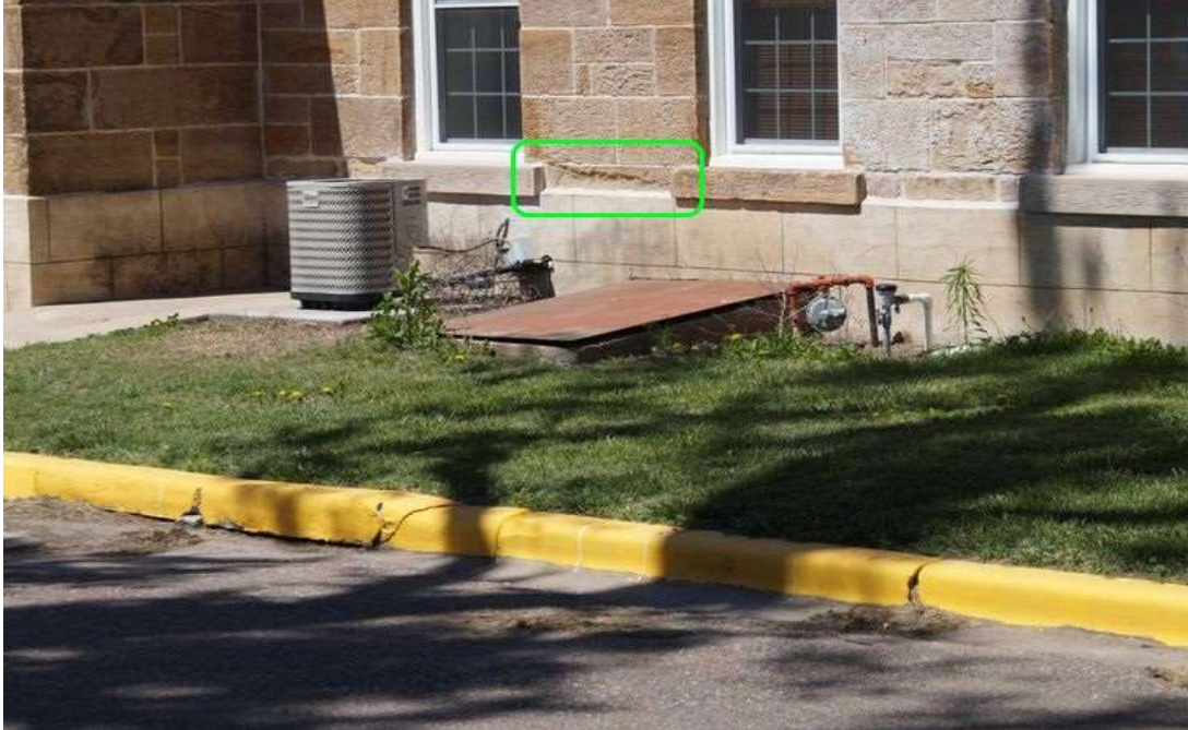
002: Old Fort Dodge Hospital ca. 1867 (KHRI: 057-1821-00004). East elevation exterior basement access; looking west-southwest. Note: spalling of the sandstone above the veneer panels is shown in the green box.
