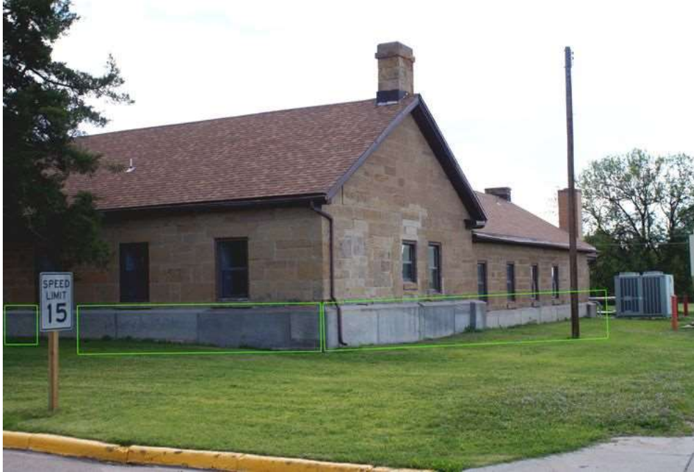
002: Fort Dodge Enlisted Men's Barracks ca. 1867 (KHRI: 057-1821-00003). South end of south barracks at the west (front) and south elevations; looking northeast. Note application of concrete/gunite at base of walls that encompasses the entire building; shown here in green.
