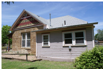
Fort Dodge - Officers House. South elevations of main building (left) and wood-framed addition (right); looking north. 05/14/2015. KSHS/Anderson, Rick.
