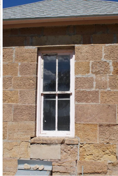
Fort Dodge – Officers House. 702 Sheridan Street. East elevation, typical 2/2, double-hung windows; looking west. 05/25/2017. KSHS/Anderson, Rick.
