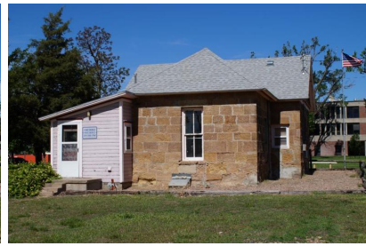
Fort Dodge – Officers House. 702 Sheridan Street. South elevations of wood-framed addition (left) and original building (right); looking west. 05/25/2017. KSHS/Anderson, Rick.
