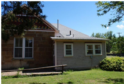
Fort Dodge - Officers House. 702 Sheridan Street. South elevation of original building (left) and wood-frame addition (right); looking north-northeast. 05/25/2017. KSHS/Anderson, Rick.
