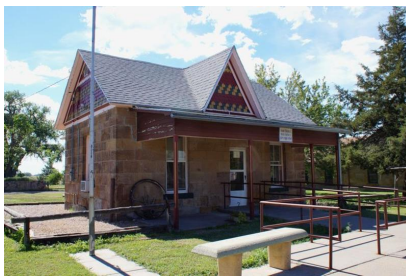
Fort Dodge - Officers House. 702 Sheridan Street. West (front) elevation; looking east. 05/25/2017. KSHS/Anderson, Rick.
