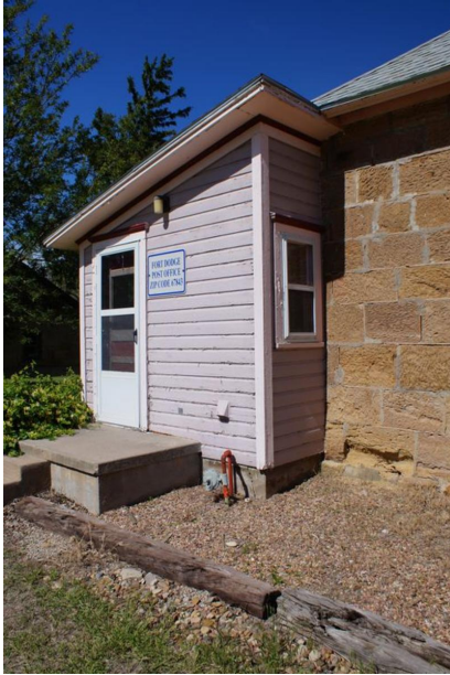
Fort Dodge – Officers House. 702 Sheridan Street. East elevation of wood-framed addition; looking southwest. 05/25/2017. KSHS/Anderson, Rick.
