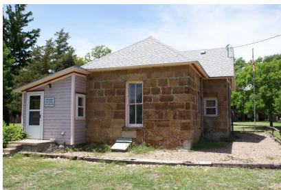
Fort Dodge - Officers House. East elevation; looking west. 05/14/2015. KSHS/Anderson, Rick.
