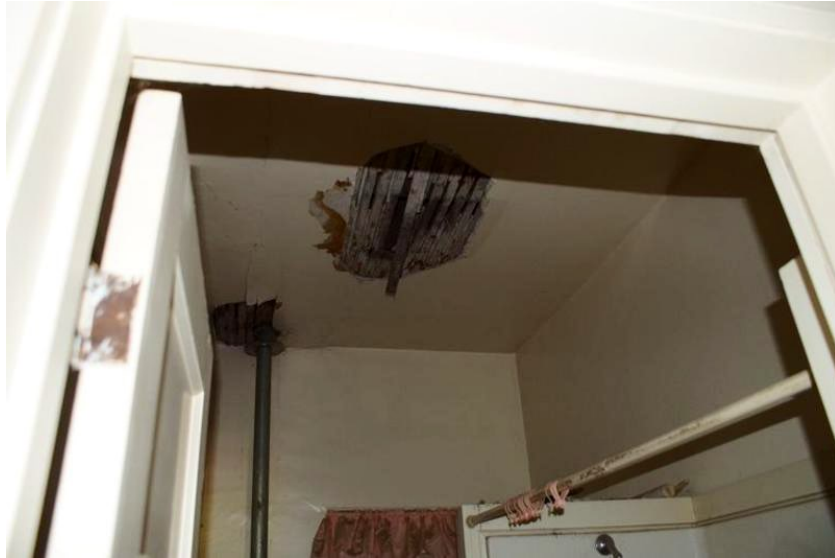
S1-009: View of plaster/lathe in ceiling
