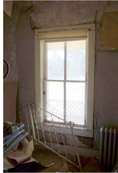
S1-010 Water entry damaging plaster & floor
