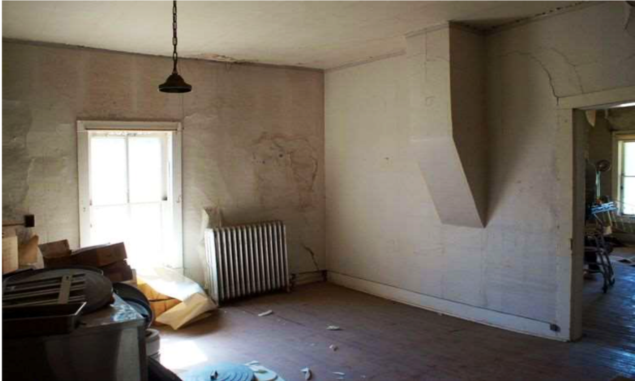
S1-007: Fort Dodge Junior Officers' Quarters ca. 1870 (KHRI: 057-1426). Interior, first-floor east half of Junior Officers Quarters; looking southeast in the northeast room. The wall with the window is the area of water intrusion. Note plaster above register and to the right of the window.
