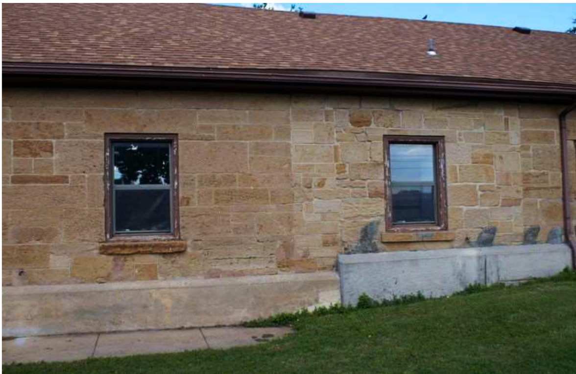
S4- 002: Fort Dodge Enlisted Men's Barracks ca. 1867 (KHRI: 057-1821-00003). South end of south barracks at the west (front) and south elevations; looking northeast. Note application of concrete/gunite at base of walls that encompasses the entire building; shown here in green.
