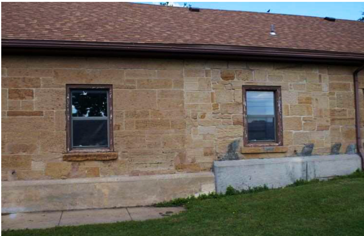
S4-004: Fort Dodge Enlisted Men's Barracks ca. 1867 (KHRI: 057-1821-00003). East elevation of south barracks; looking west. Note two different applications of concrete/gunite to lower areas of the walls.
