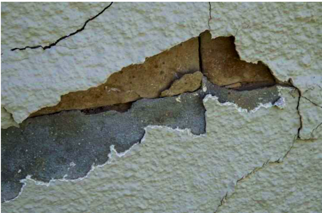
S3-002: Fort Dodge Army Quartermaster Building ca. 1867 (KHRI: 057-1399). West elevation; looking east. Note the application of concrete first under the second attempt with stucco.
