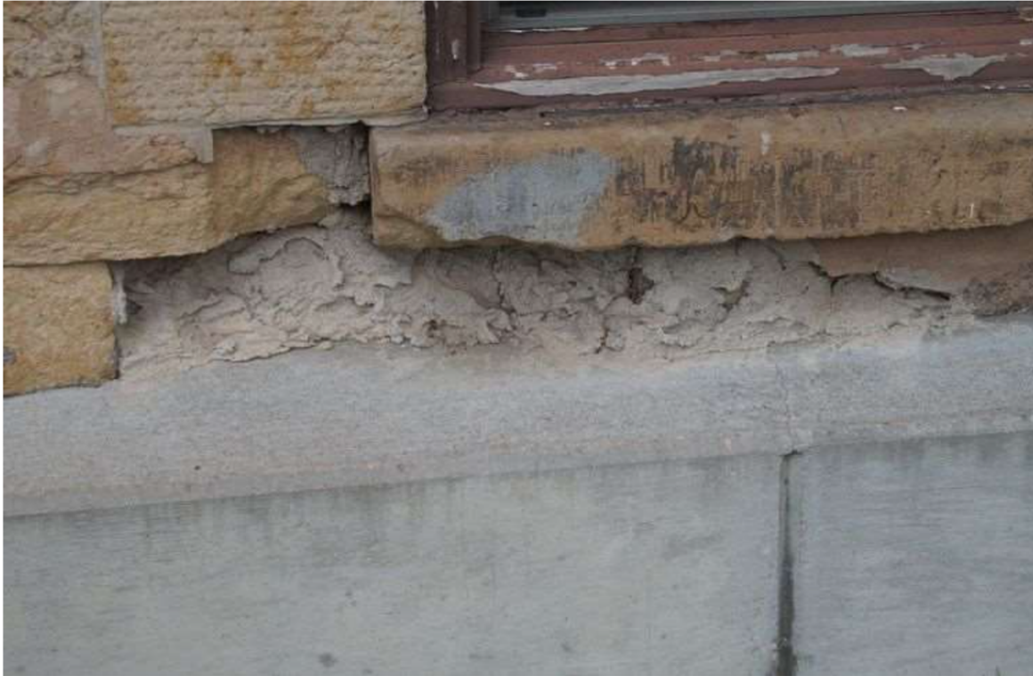
S4-005: Fort Dodge Enlisted Men's Barracks ca. 1867 (KHRI: 057-1821-00003). South barracks east elevation, typical window sill and spalled sandstone just above the concrete/gunite; looking west.
