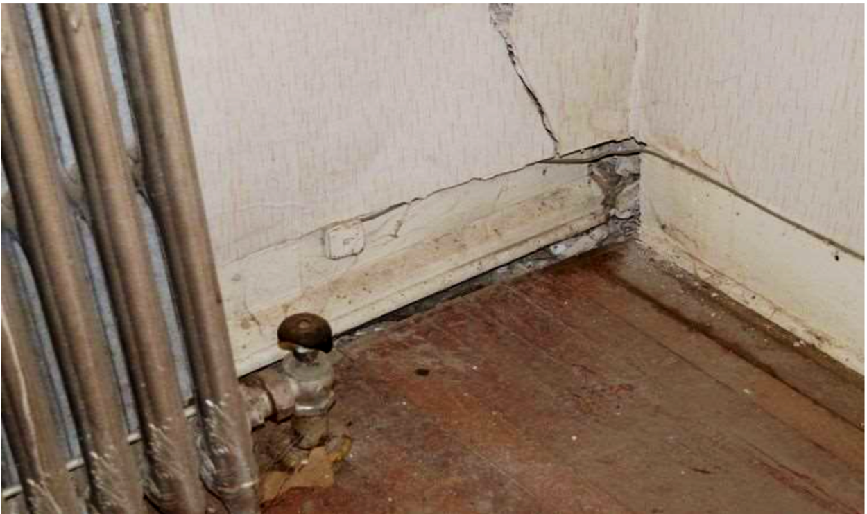
S1-008: Fort Dodge Junior Officers' Quarters ca. 1870 (KHRI: 057-1426). First-floor, east side of Junior Officers Quarters; water damage and settling of the floor from the wall in the northeast corner of the northeast room.
