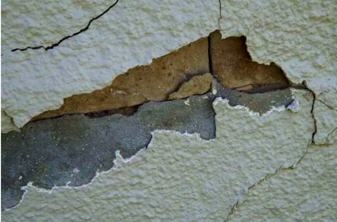
S3-004: Fort Dodge Army Quartermaster Building ca. 1867 (KHRI: 057-1399). East elevation at southeast corner of building; looking west. Note bottom corner stone has totally spalled.
