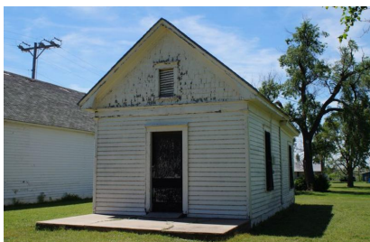
Fort Dodge - Dead House (Relocated). 317 Pershing Street. North (front) and west elevation; looking south-southwest. 05/25/2017. KSHS/Anderson, Rick.
