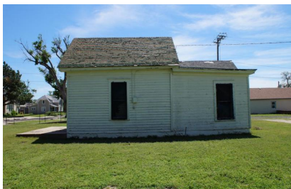
Fort Dodge - Dead House (Relocated). 317 Pershing Street. West elevation of the original building (left) and shed addition (right); looking north-northeast. 05/25/2017. KSHS/Anderson, Rick.
