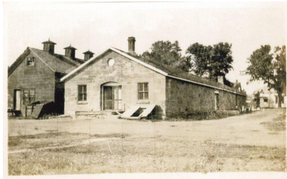
Fort Dodge – Army Quartermaster Building. 217 Pershing Street. South and east elevations; looking northwest. 1916. Image courtesy of Heather Douglas and Joanne VanCoevern. August 2017. KSHS/Anderson, Rick.
